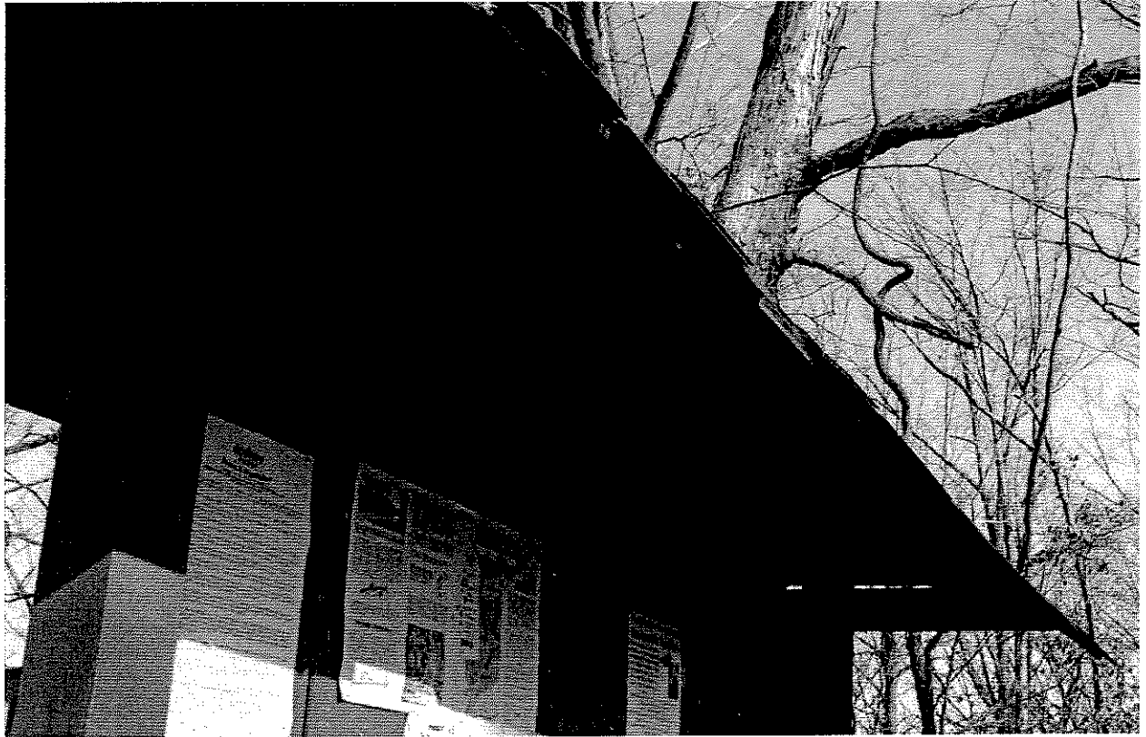
Figure10 , Underside of the kiosk roof
